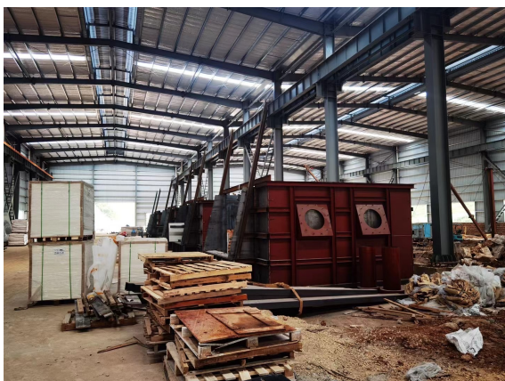
Melting furnace insulation
